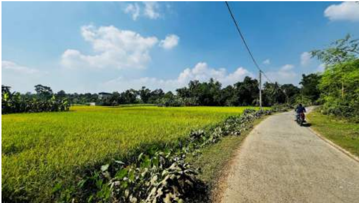
Image 10: Road connecting the Protected Monument to Harua Road.
