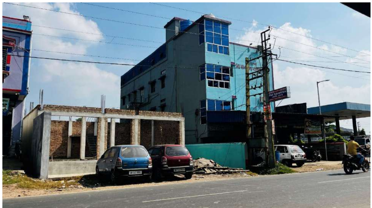
Image 14: View of A Nursing Home and adjoining filling station towards North in Regulated Area.
